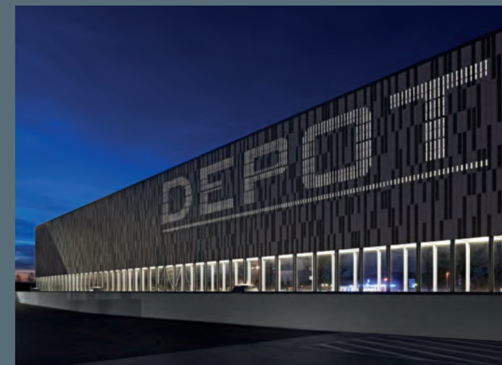
DEPOT noise protection wall, Niedernberg Lighting Design: studiocandela, Herford
